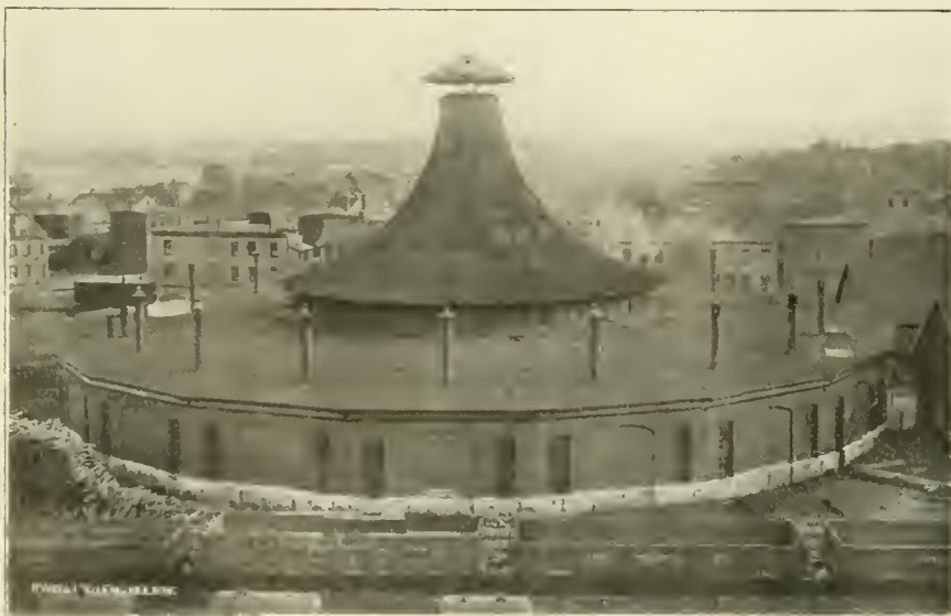
OLD FASHIONED ROUNDHOUSE AT MONCTON, N. B., WITH HIGH, CONE-SHAPED VENTILATOR—INTERCOLONIAL RAILWAY OF CANADA—NOW REPLACED BY A MODERN SHOP.
